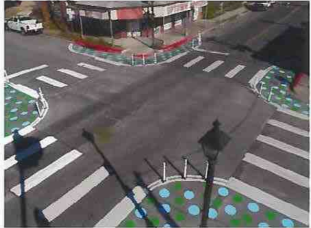
Utilizing paint and temporary bollards to test curb bulb-outs
