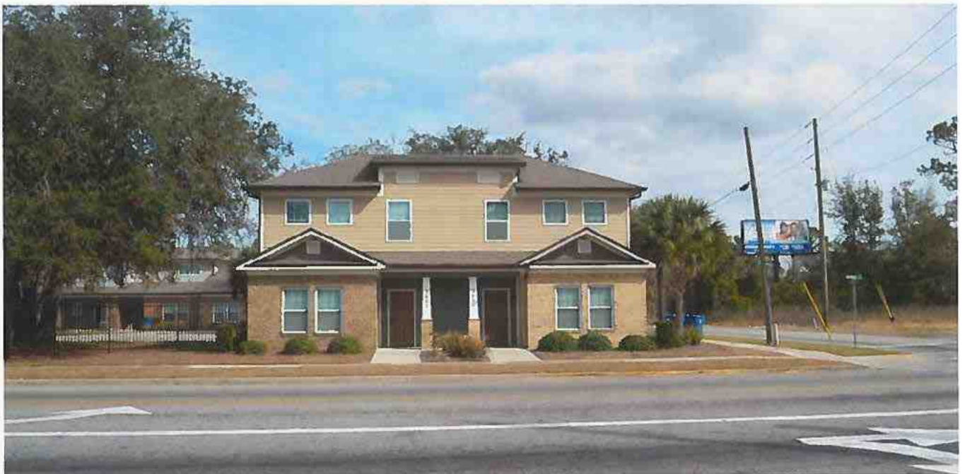
New development of housing at Norwich Commons
