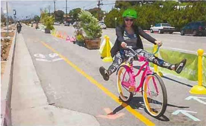
Above: images of testing street changes with temporary paint; a pop-up bike boulevard using cones and planters.
