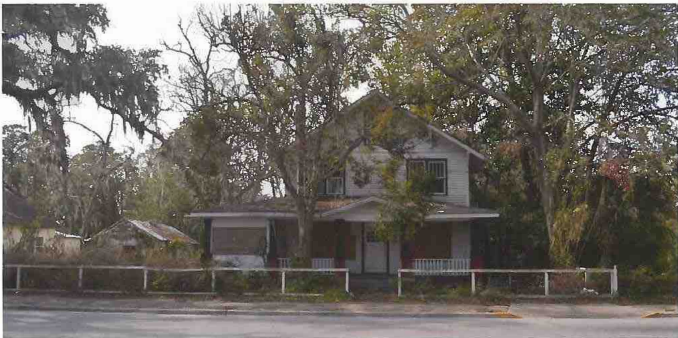
Housing in need of repair or redevelopment along Norwich Street
